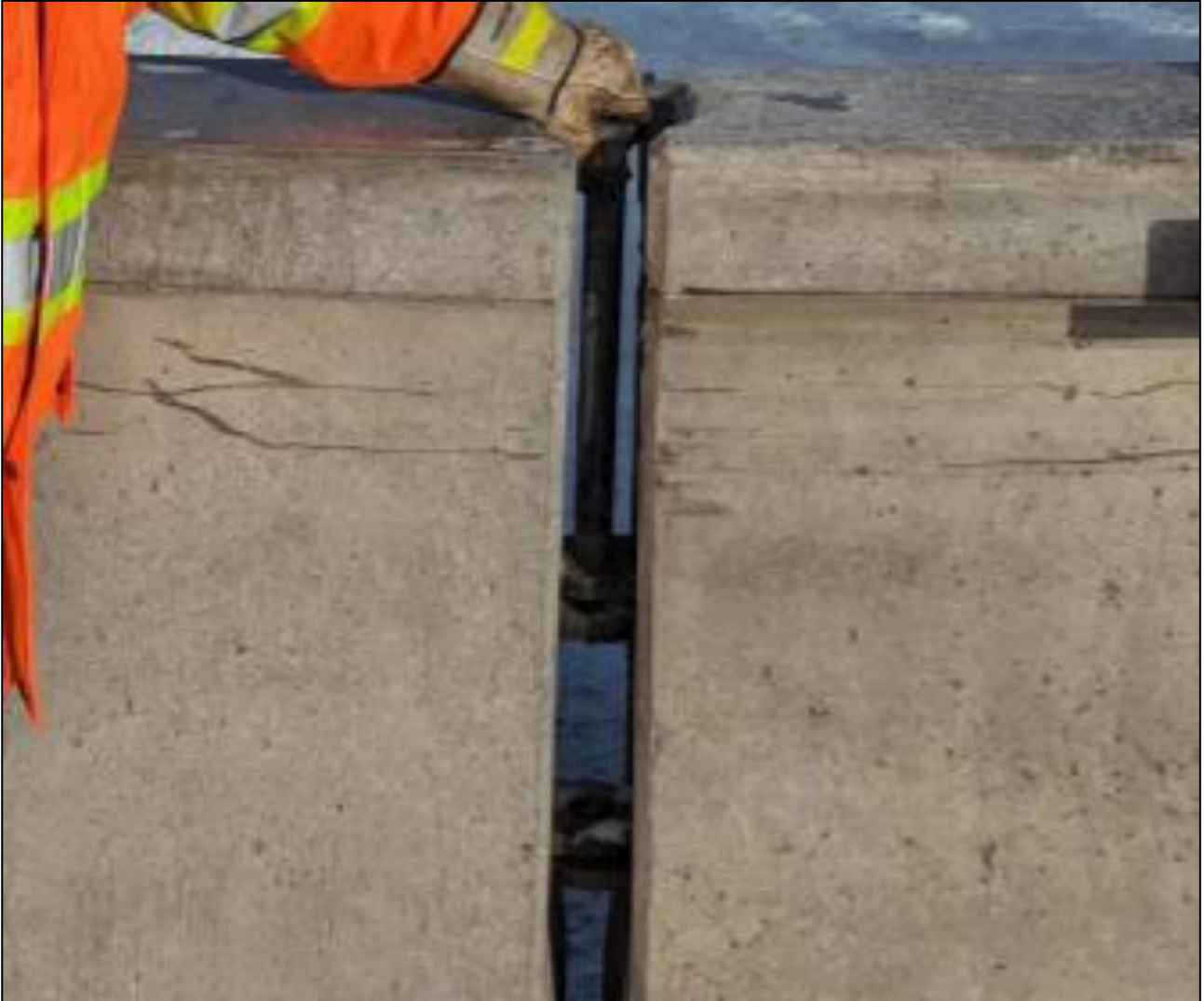
Figure 6: Insertion of Connecting Pin
