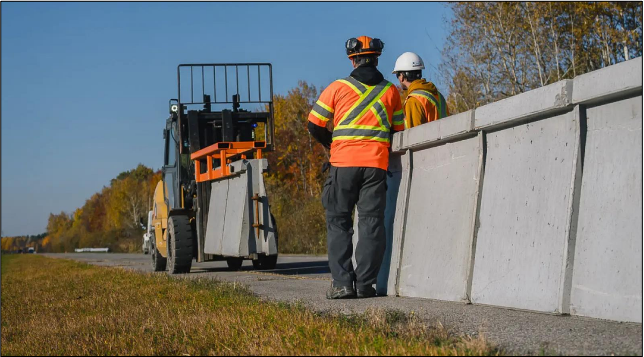
Figure 1: Forklift Handling of TALL42™ Units
