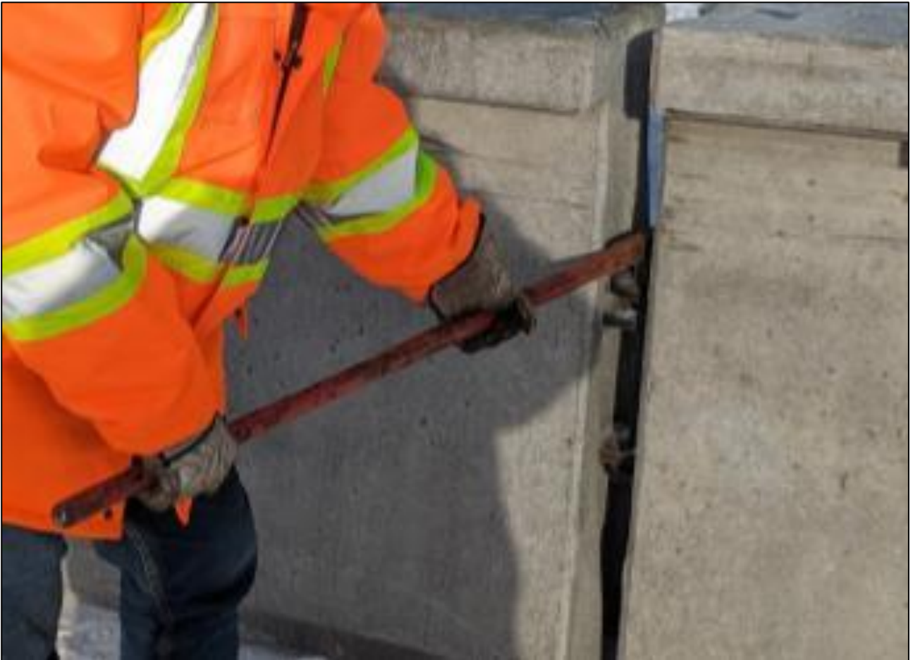
Figure 7: Using a Pry Bar to Adjust Barrier Alignment
