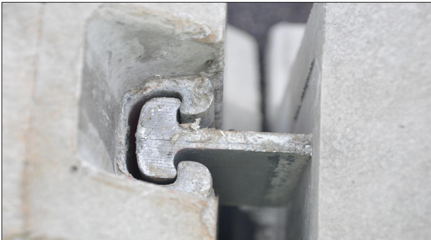
Figure 18: T-Coupler and Y-Coupler Assembly
