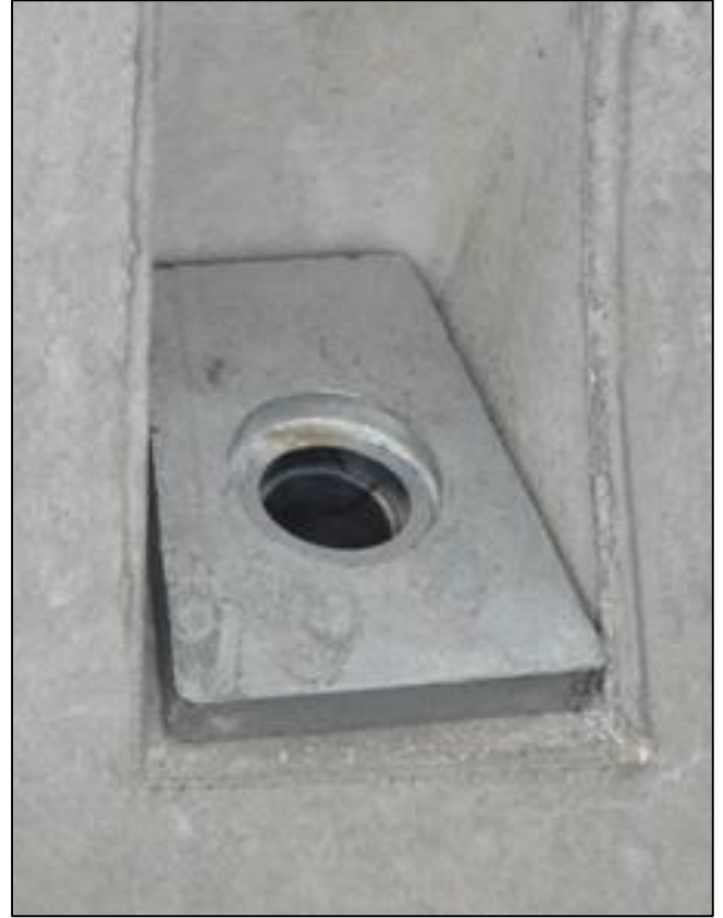
Figure 21: Placement of the Square Washer
