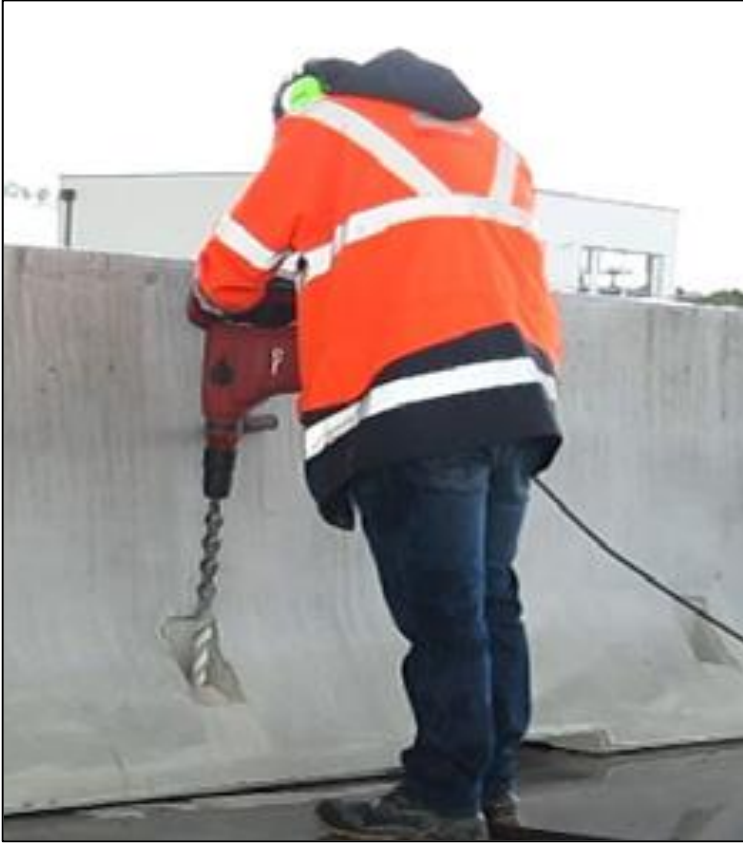
Figure 20: Drilling Anchor Holes
