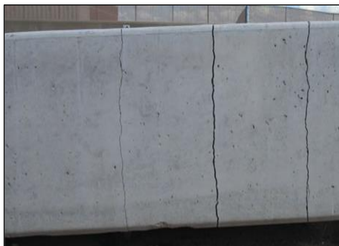
Figure 25: Unacceptable Vertical Cracking
