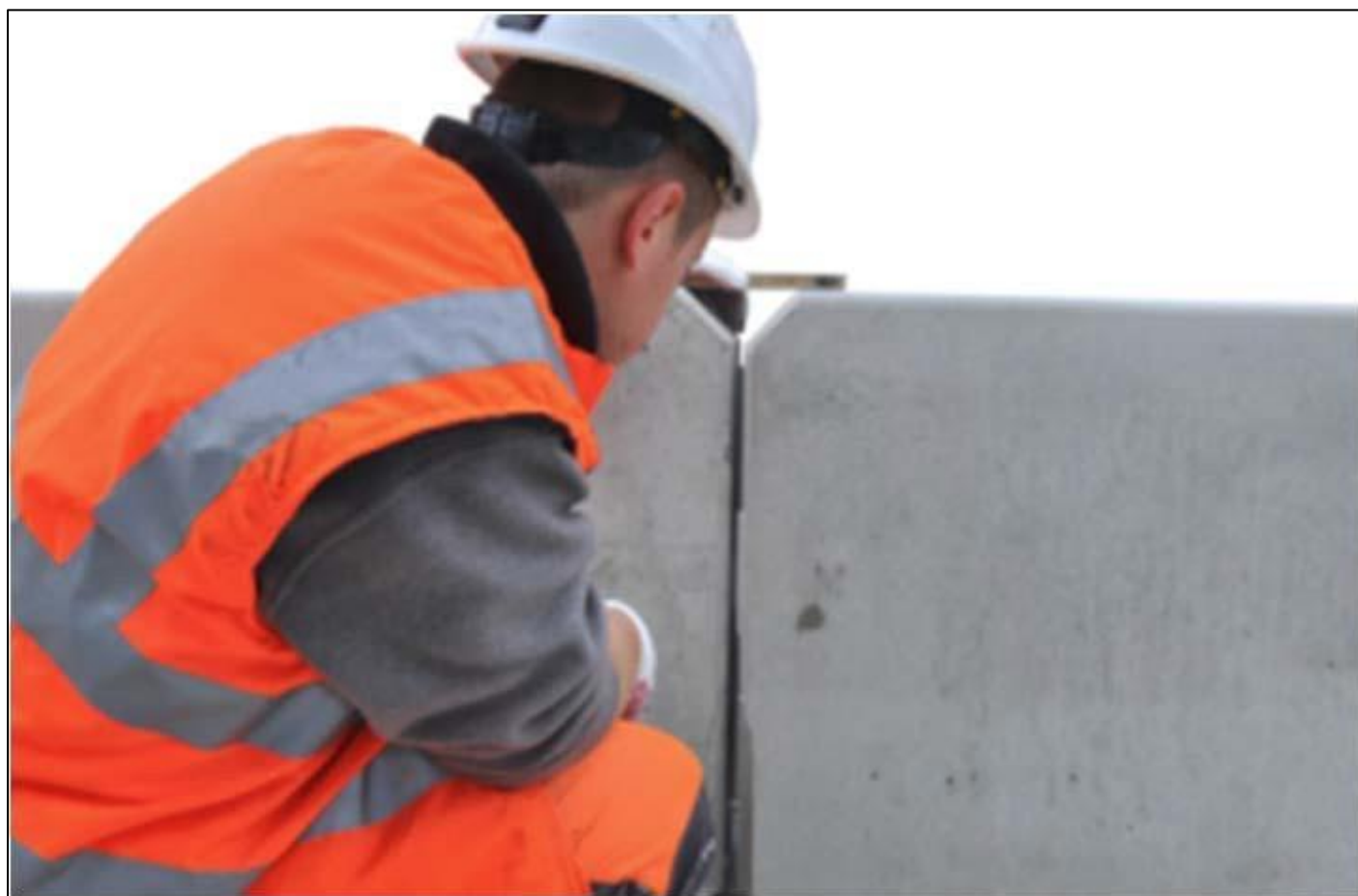
Figure 19: Inspection of Height Alignment
