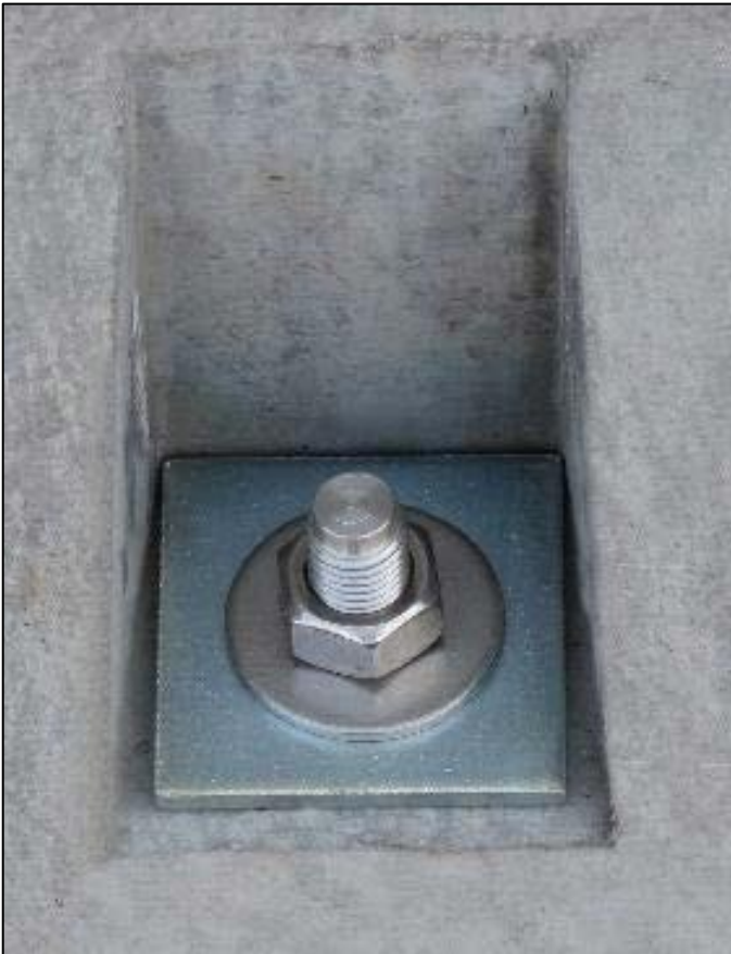
Figure 22: M20 Threaded Rod Anchoring
