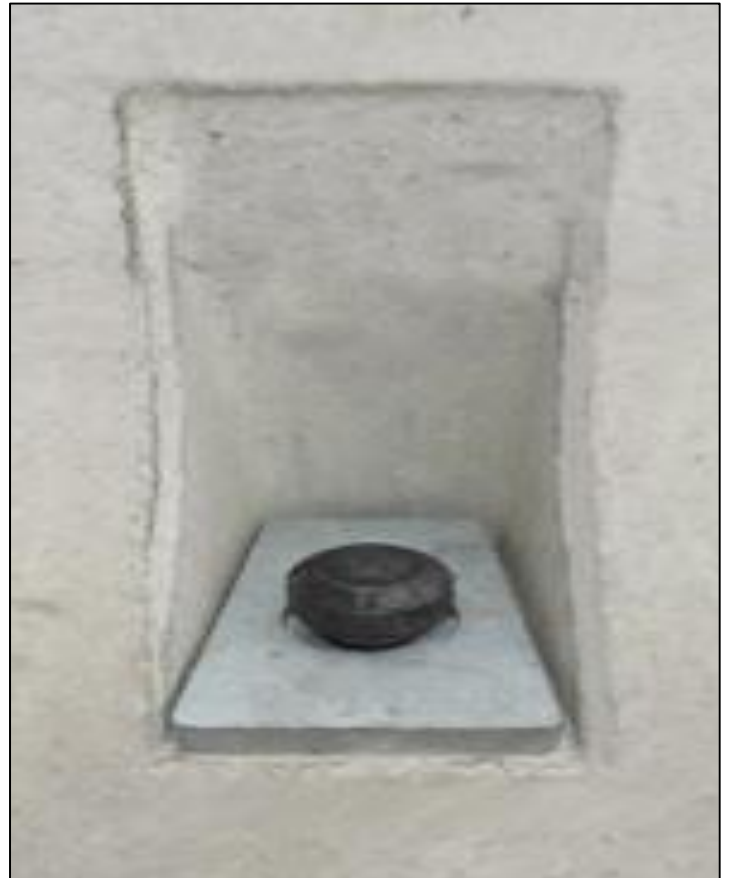
Figure 23: M25 Pin Anchoring
