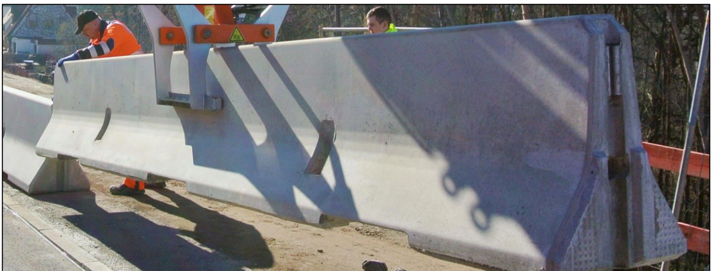
Figure 17: Aligning Barriers
