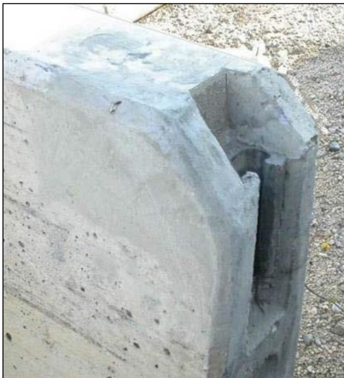
Figure 25: Repair of Y Profile
