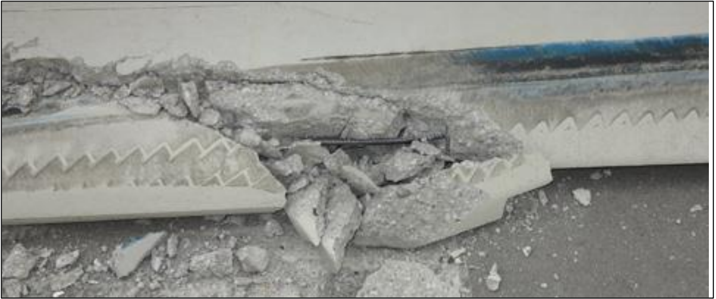
Figure 21: Spalling Exposing Rebar
