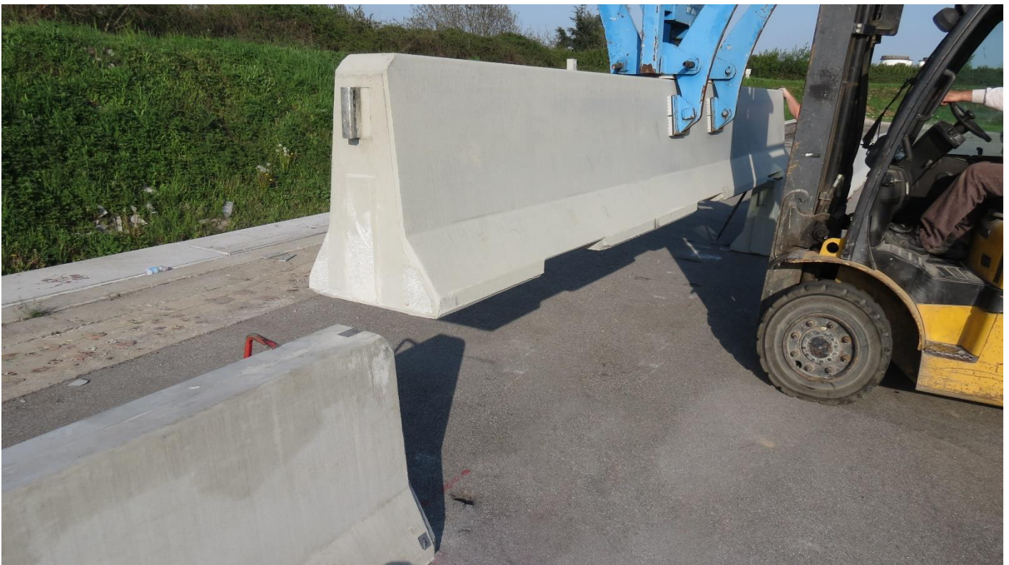
Figure 16: Aligning Barriers
