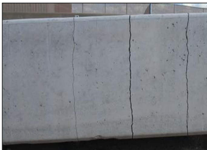
Figure 20: Unacceptable Vertical Cracking
