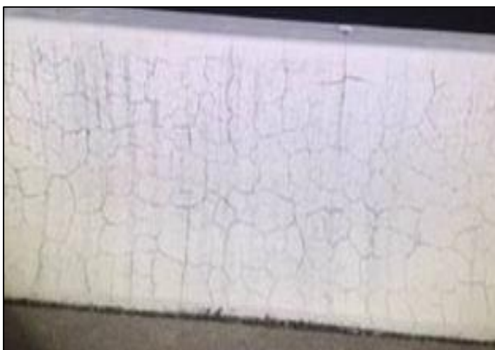
Figure 19: Acceptable Hairline Cracks
