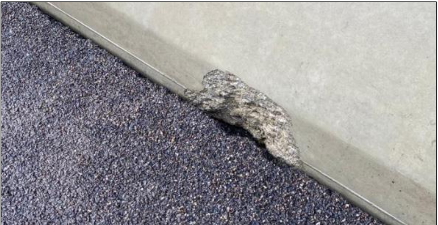
Figure 22: Spalling with no Exposure of Rebar
