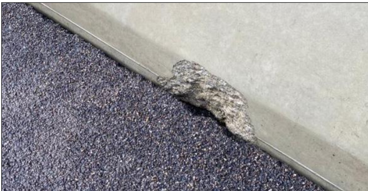
Figure 23: Spalling with no Exposure of Rebar
