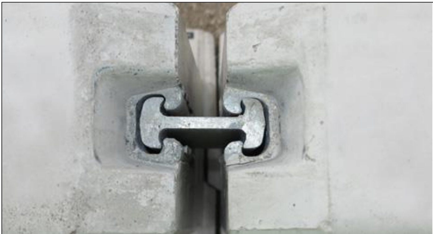
Figure 17: Coupler Assembly
