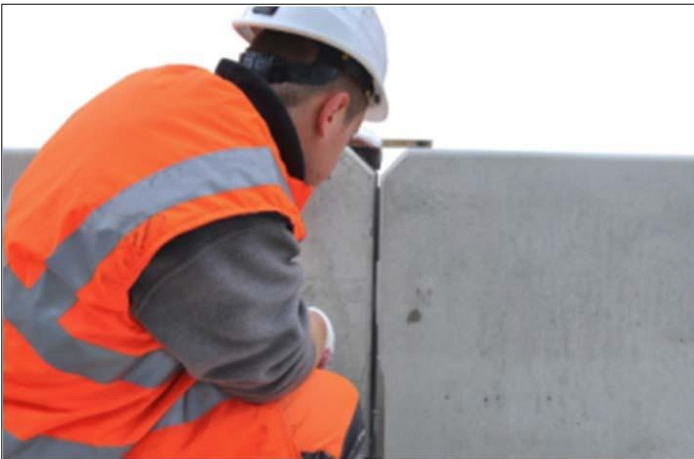
Figure 18: Inspection of Height Alignment
