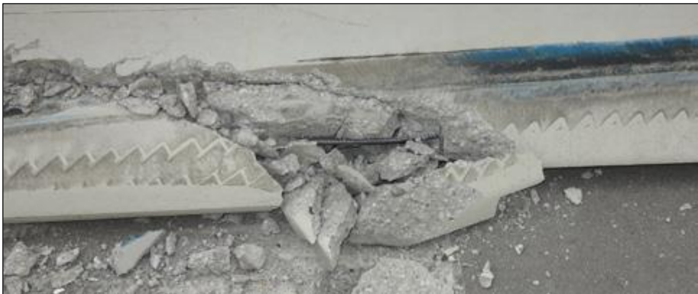
Figure 22: Spalling Exposing Rebar
