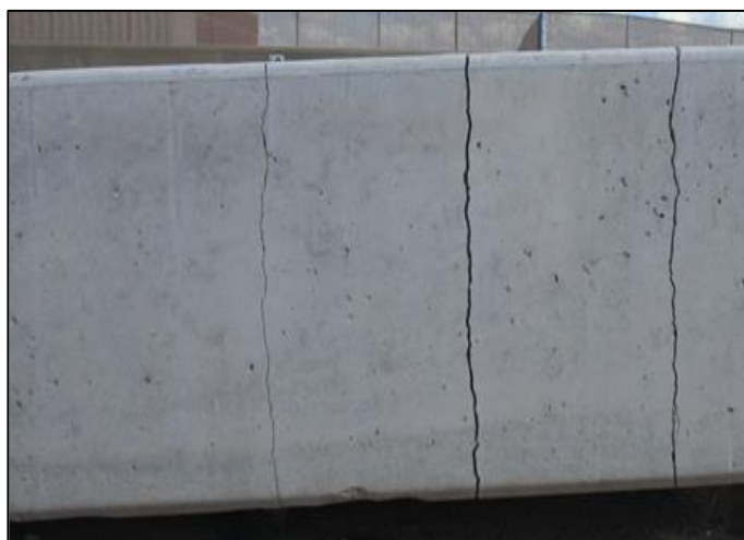
Figure 21: Unacceptable Vertical Cracking
