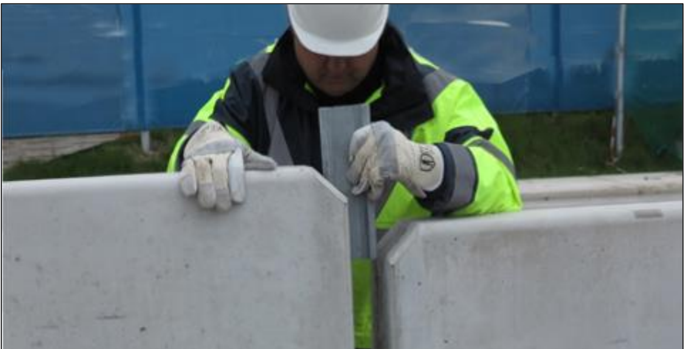
Figure 16: Insertion of Coupler
